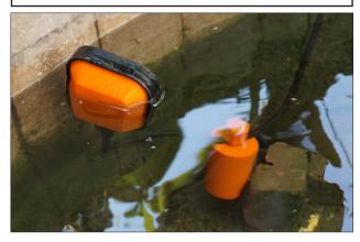
Float switch in 'minimum water level' position. Pump turns on.
